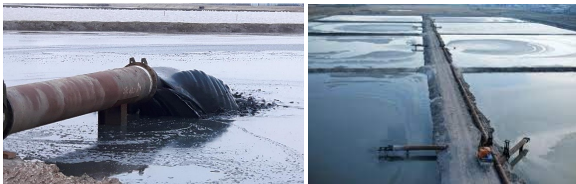
Figure 20 Filling of pilot site 'Kleirijperij' with dredged sediment
