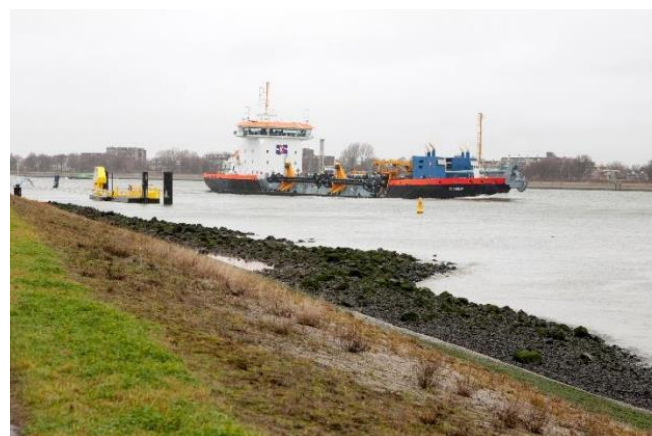
Figure 4. Hydraulic Dredger Ecodelta at the Reallocation Site
