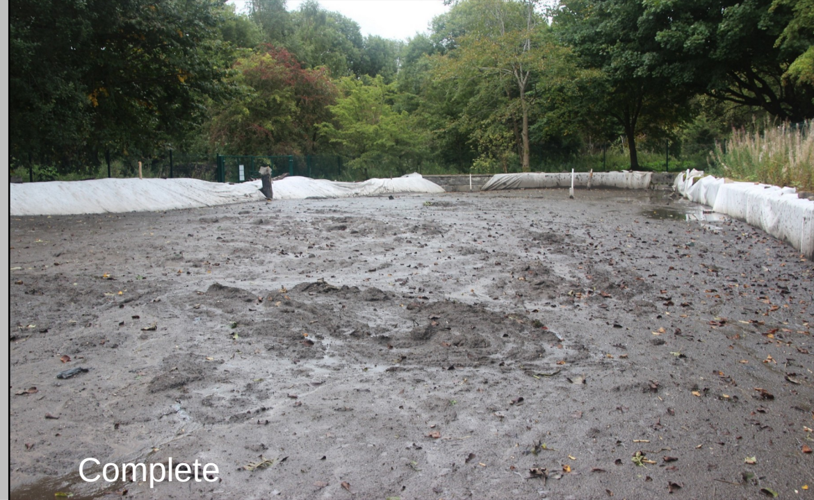
Basin lined with geofabric and wells installed
