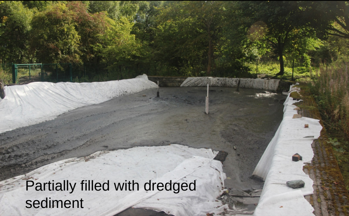
Earthworks to create basin
