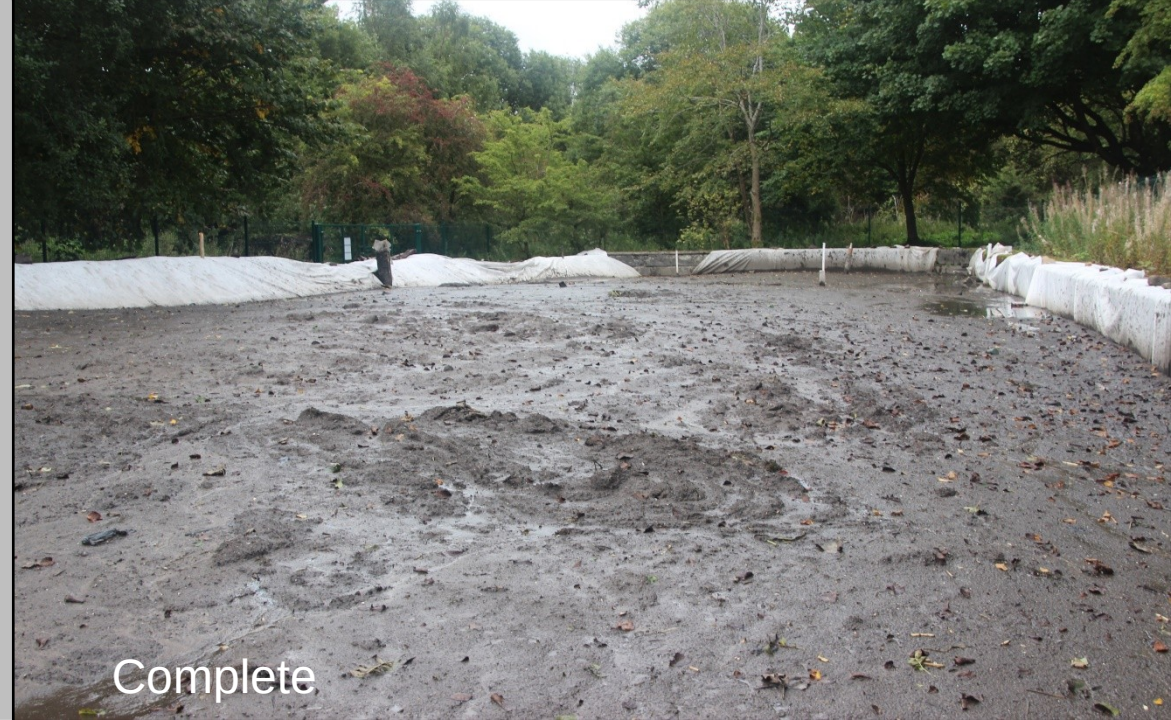
Basin lined with geofabric and wells installed
