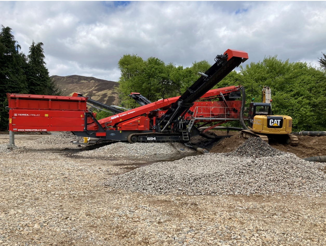
Screening to remove cobbles and gravel
