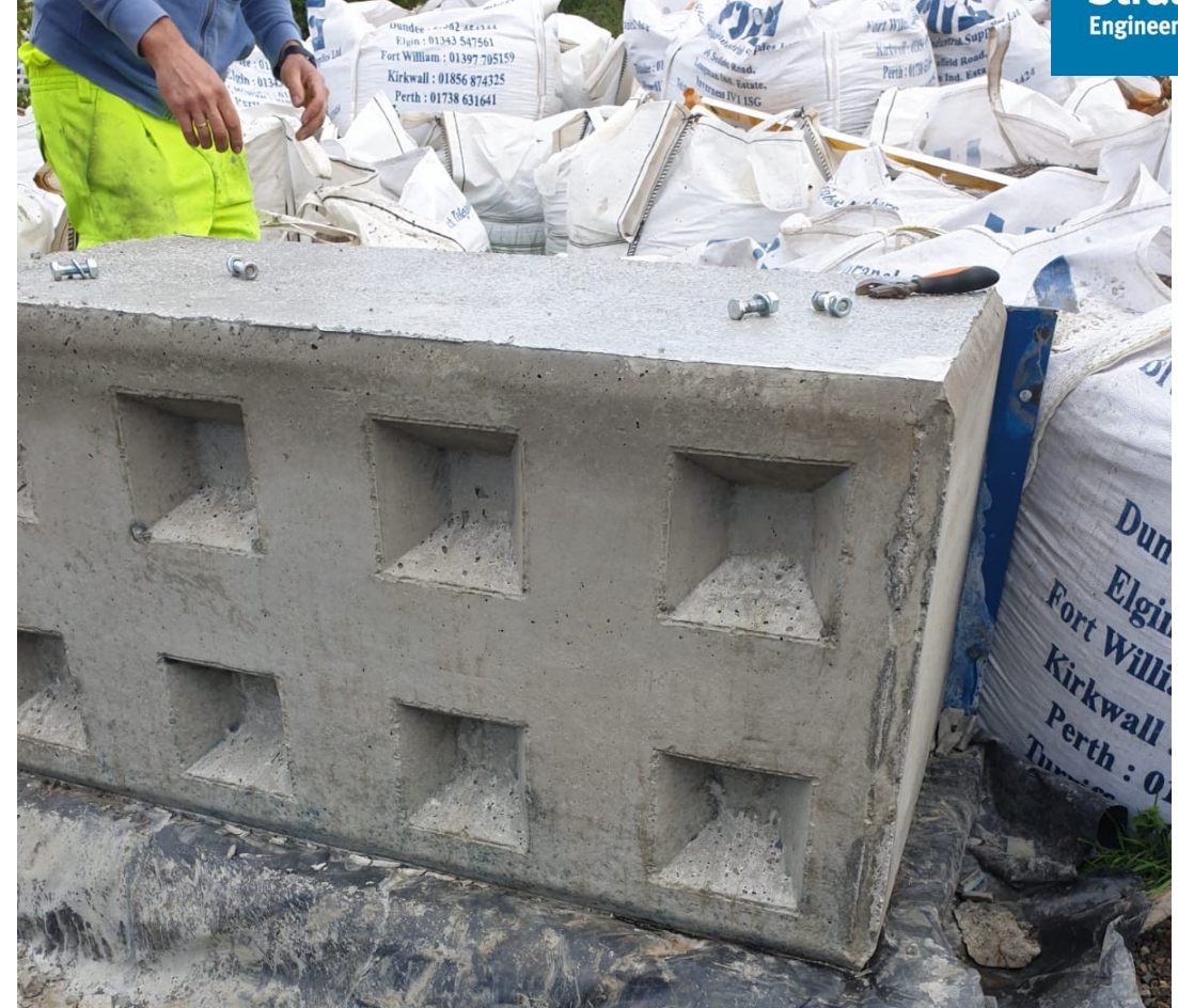
1600mm long concrete 'lego' block
