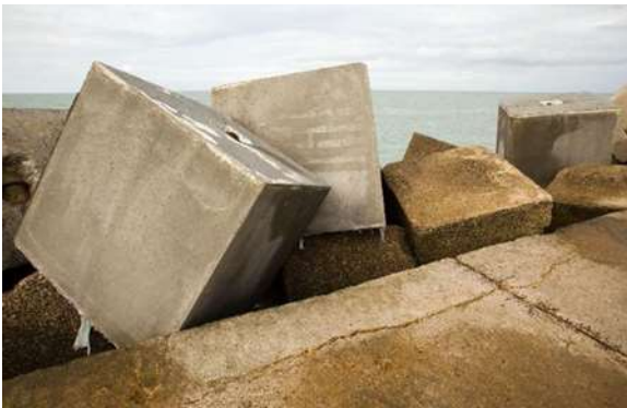
Sediment used in concrete for coastal defense blocks. SEDIMATERIAUX, port of Dunkirk
