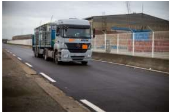
Sediment used in harbour road base. SEDIMATERIAUX, Ibid.
