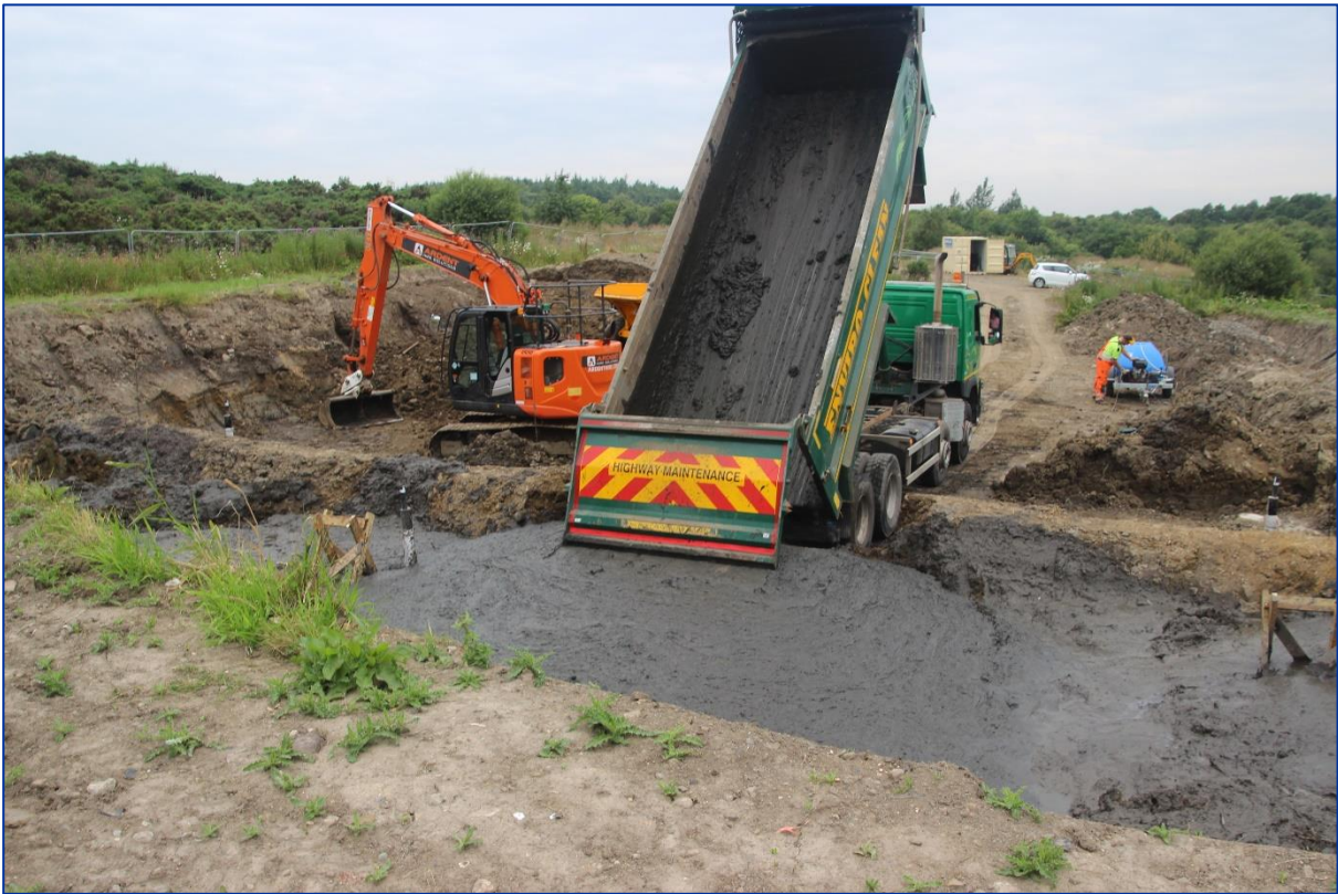
Figure 23. Dredged sediment being dumped into Cell F1.
