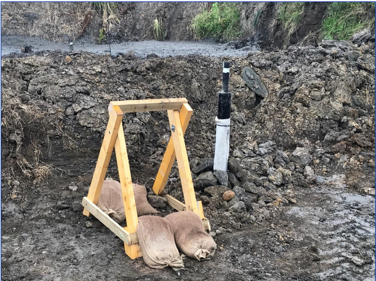
Figure 32. Well MW7 with A-frame anchored using sand bags.
