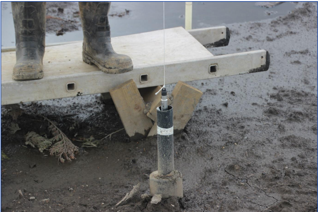
Figure 44. TD-Diver® water level logger being installed in MW5.
