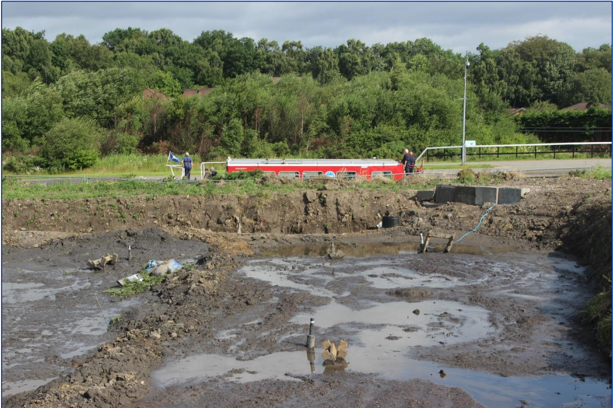
Figure 34. Cells F1 and F2 with canal barge.
