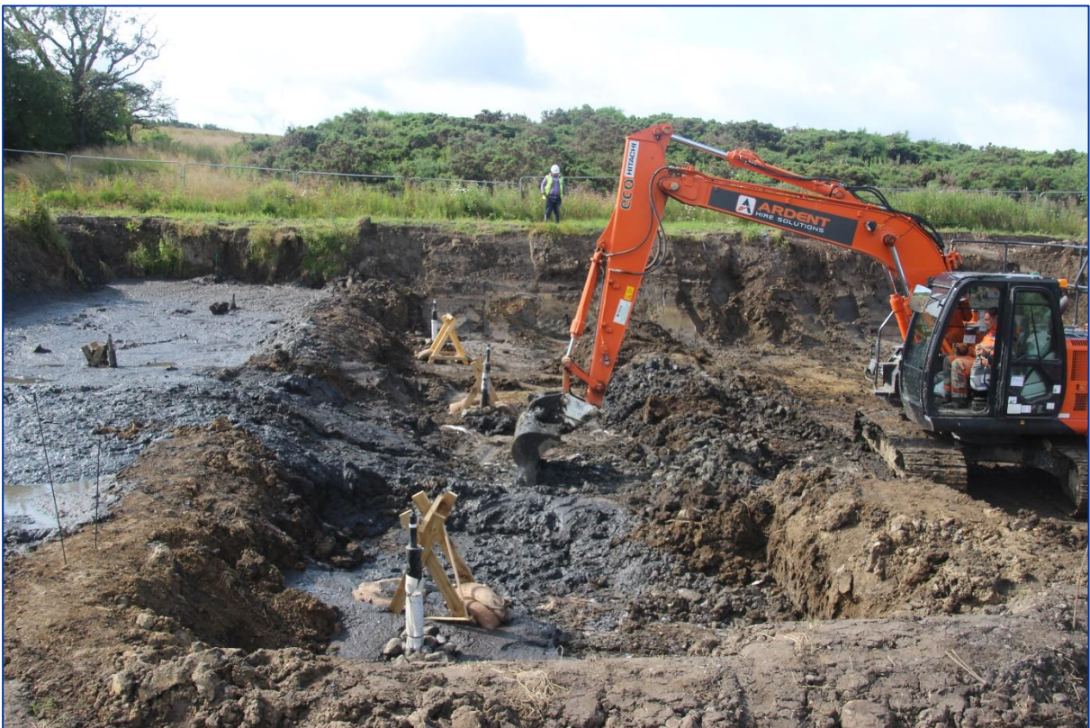
Figure 28. Cell F2 after first load of dredged sediment.
