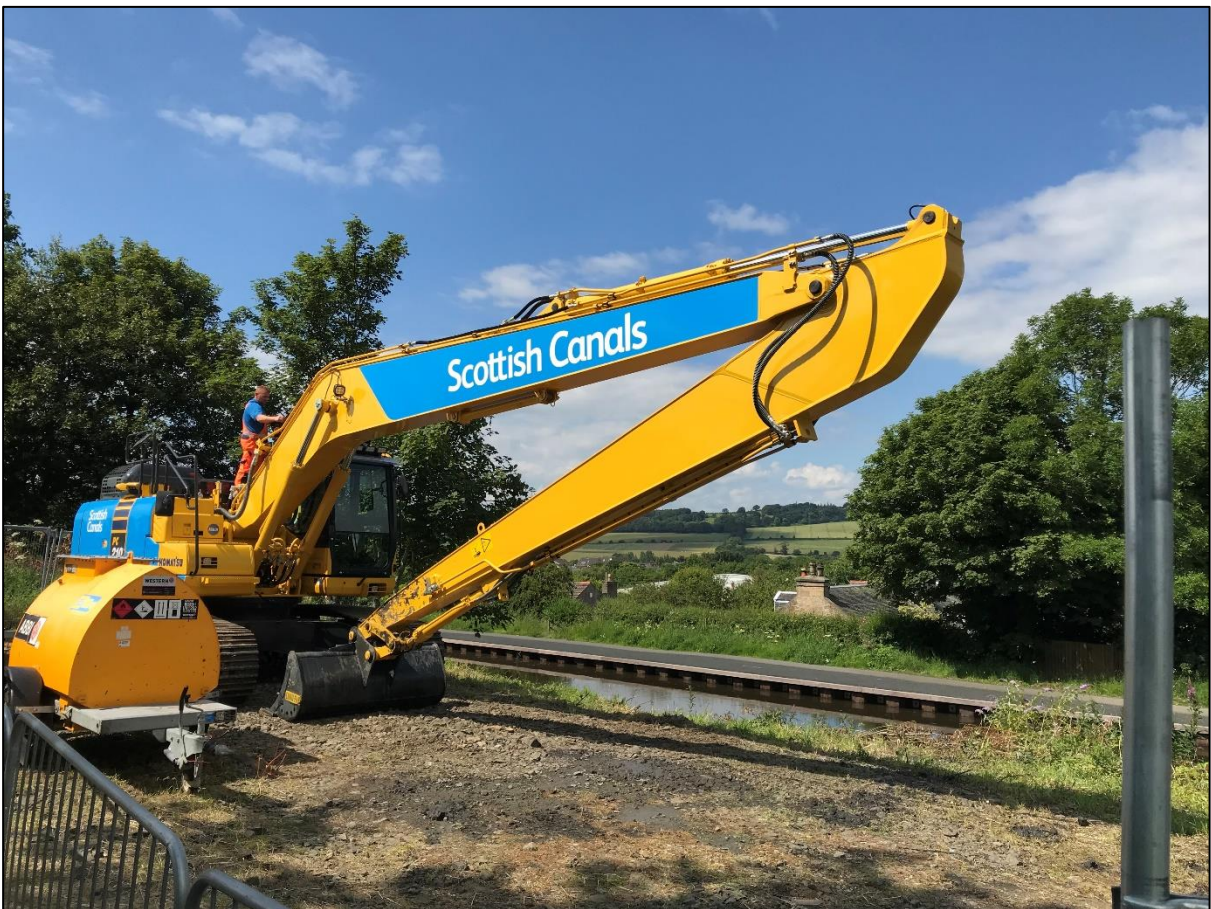
Figure 16. Long-reach excavator used to unload sediment from the barge at Linlithgow.
