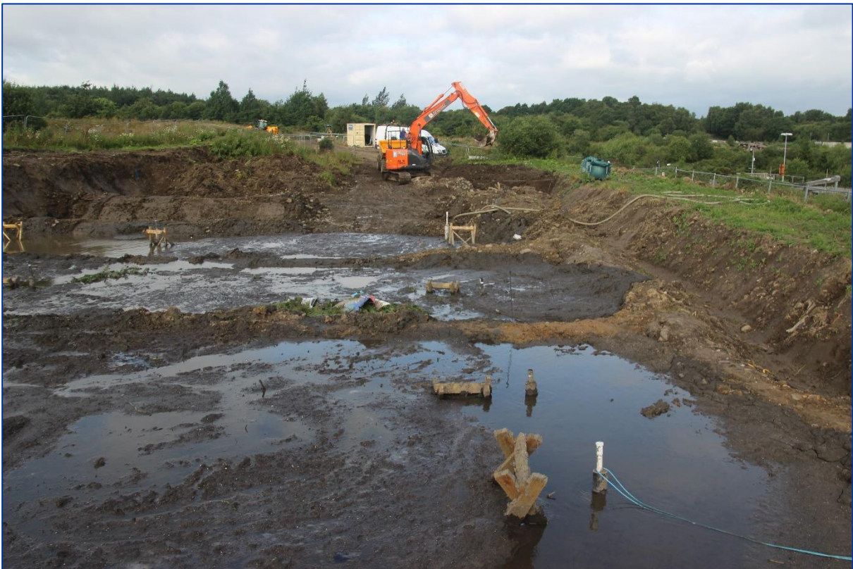
Figure 30. Cells F1 and F2 showing surface water on top of sediment.
