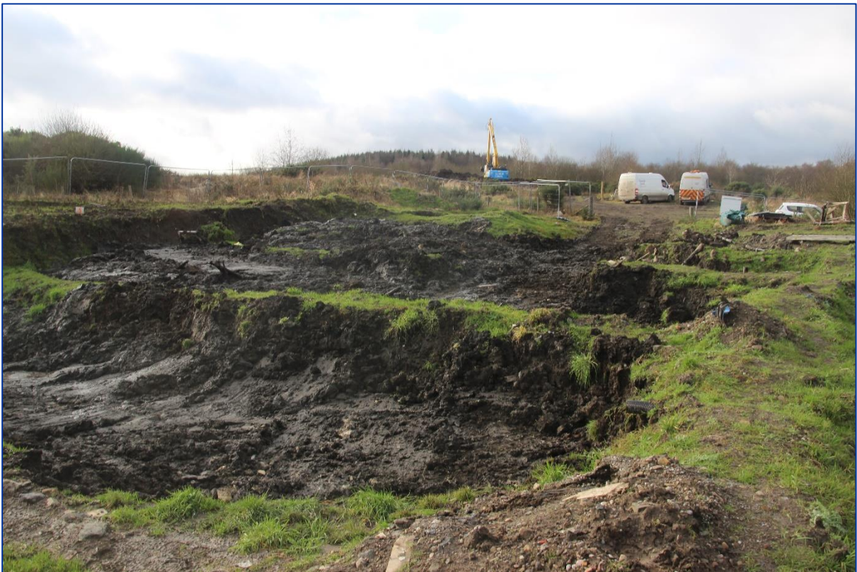
Figure 50. Excavation of material from cell F3 and F4, January 2020.
