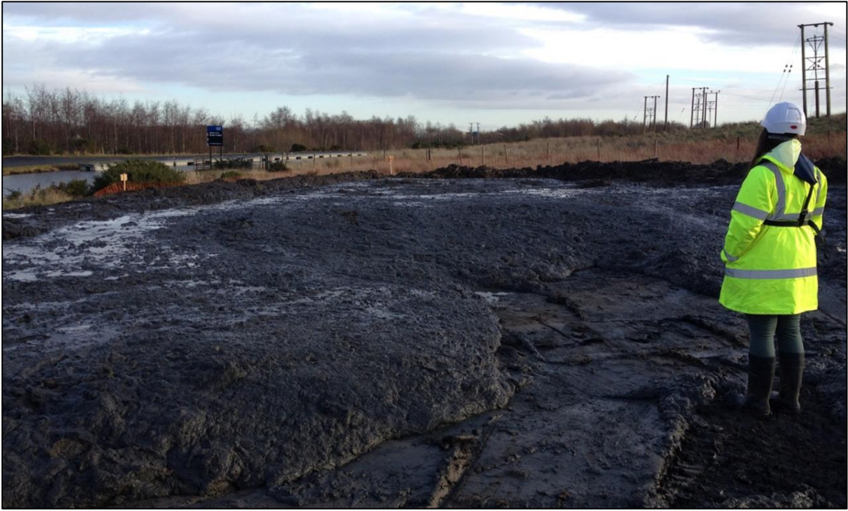
Figure 13. Photograph showing placement of dredged sediments in 2017.
