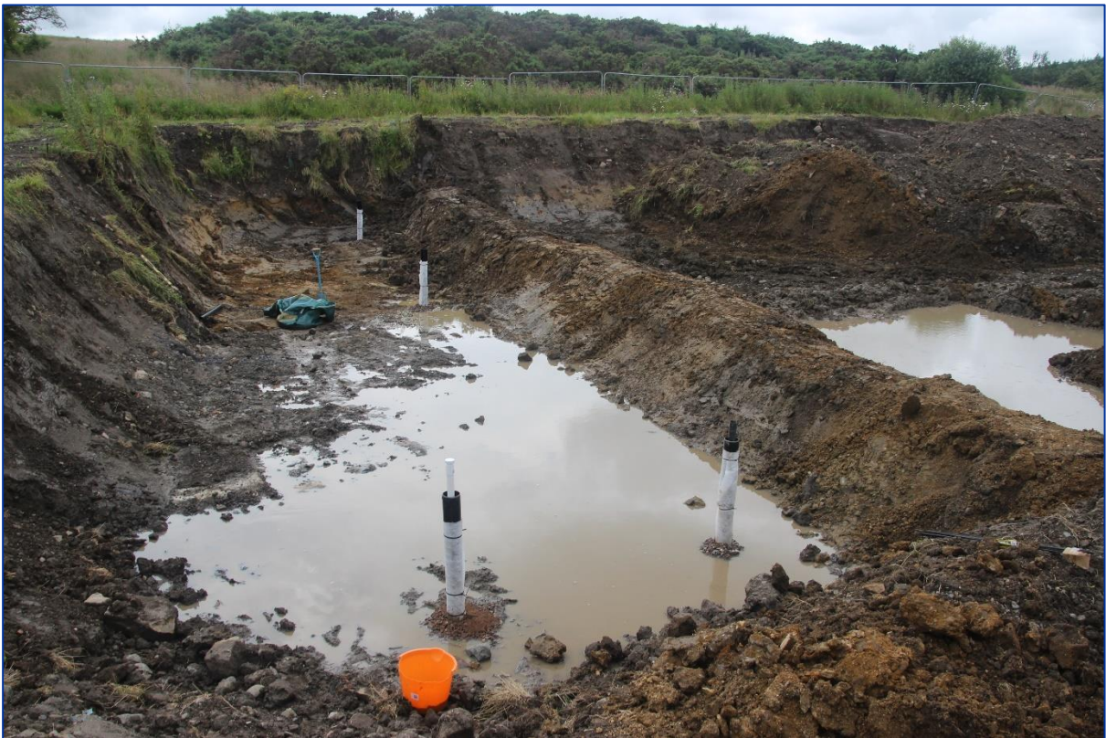
Figure 20. Cell F1 with monitoring wells in position ready for sediment.
