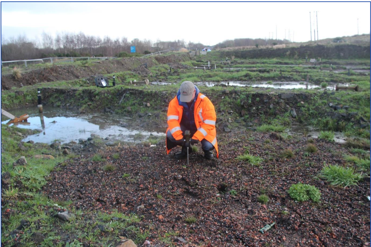
Figure 48. Using the MEXE cone penetrometer to determine soil strength in cell F6.
