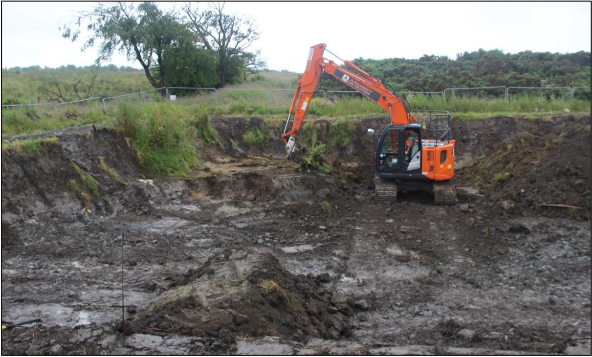
Figure 17. Excavation of the cells prior to sediment deposition.
