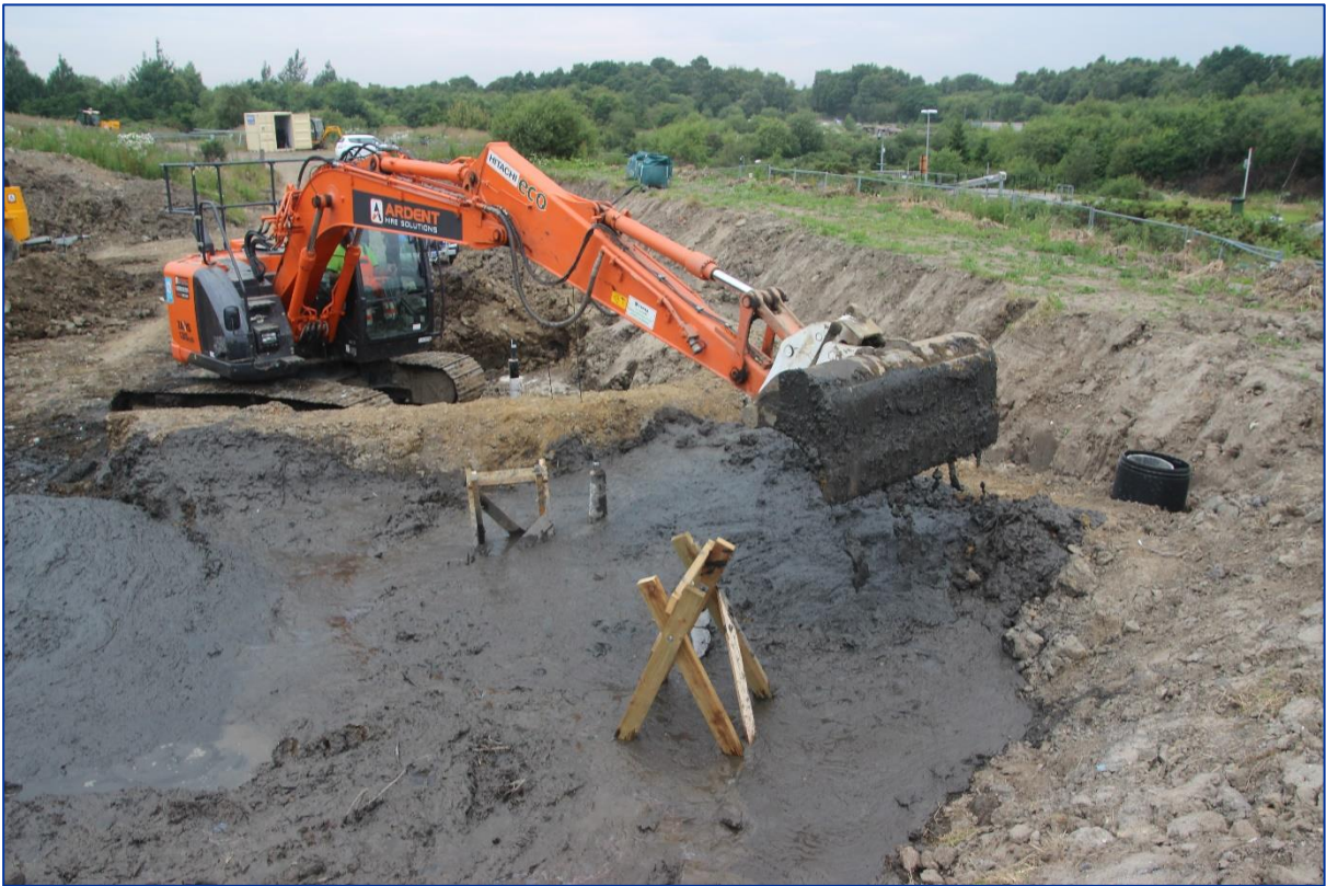
Figure 25. Loader redistributing sediment within cell F1.
