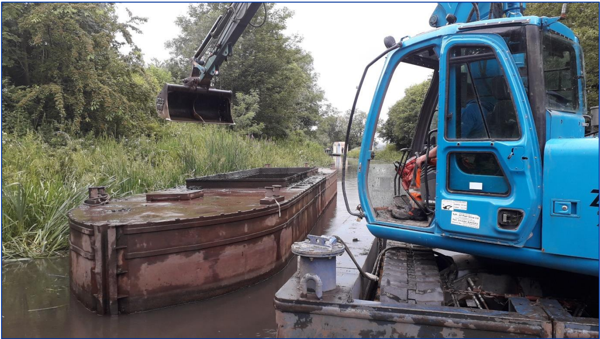
Figure 15. Dredging on the Union Canal at Linlithgow.
