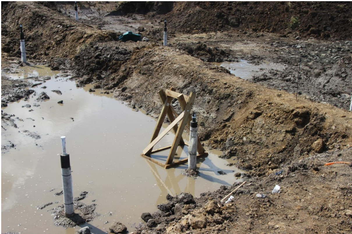
Figure 22. MW01 and MW02 in cell F2 showing A-frame in position.
