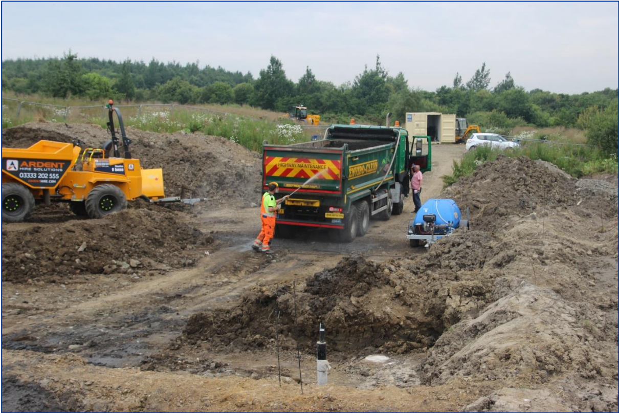
Figure 29. Tipper lorry being cleaned using a power washer after sediment delivery.
