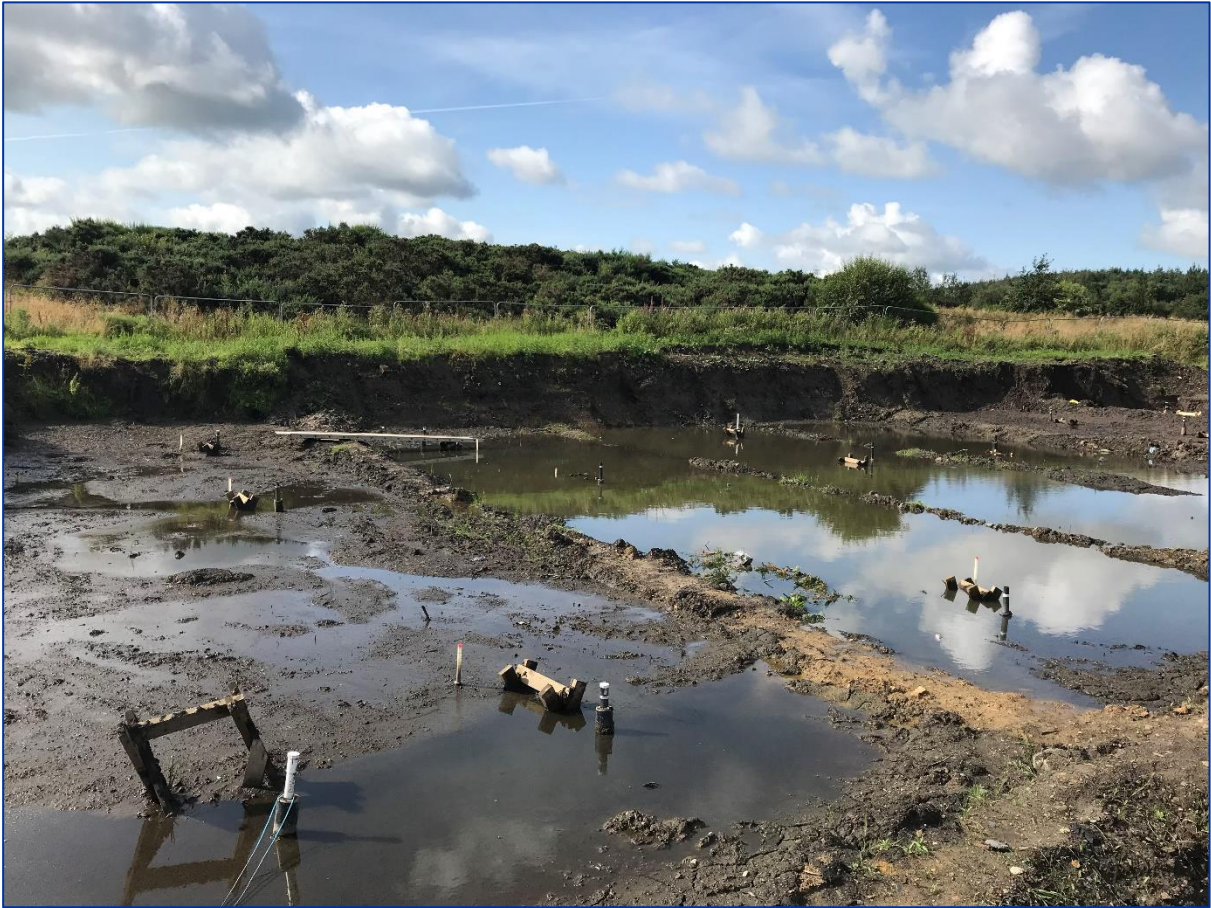
Figure 37. Site on August 12, 2019 after heavy rain during the previous weekend.
