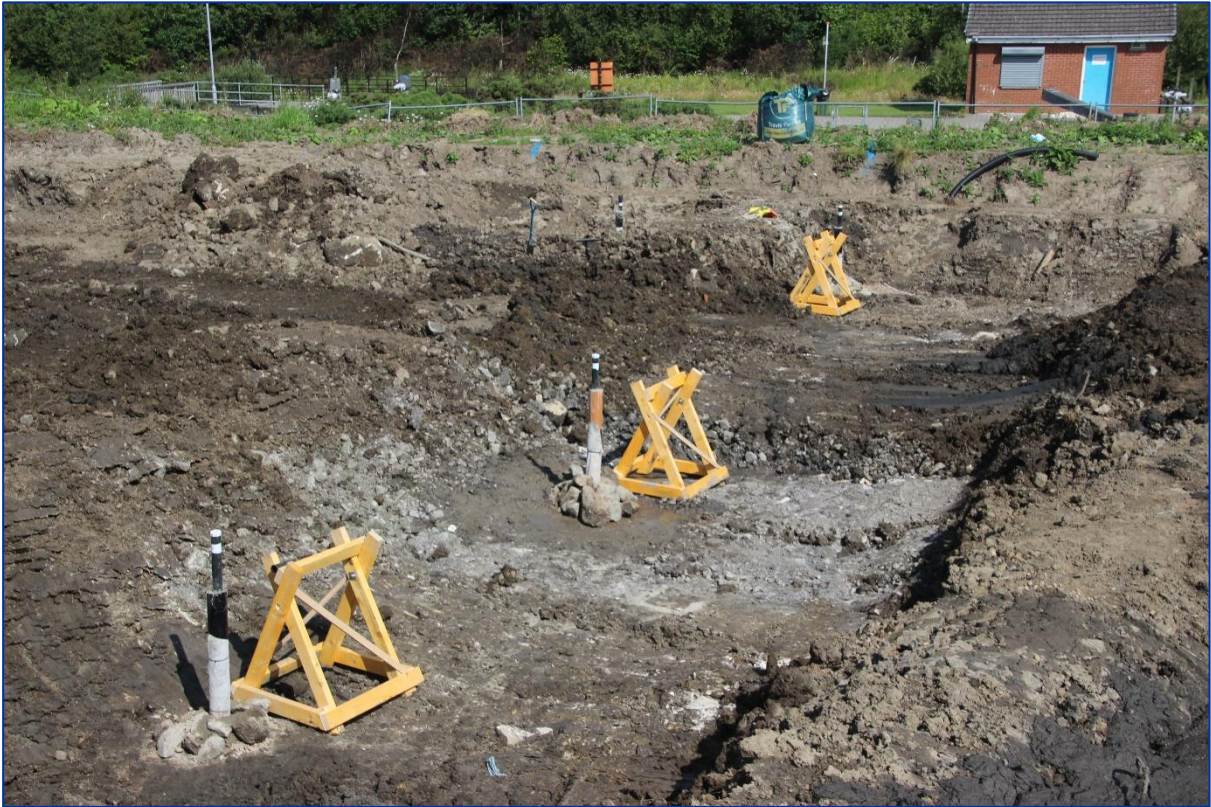
Figure 35. Cell F3 prior to sediment addition.
