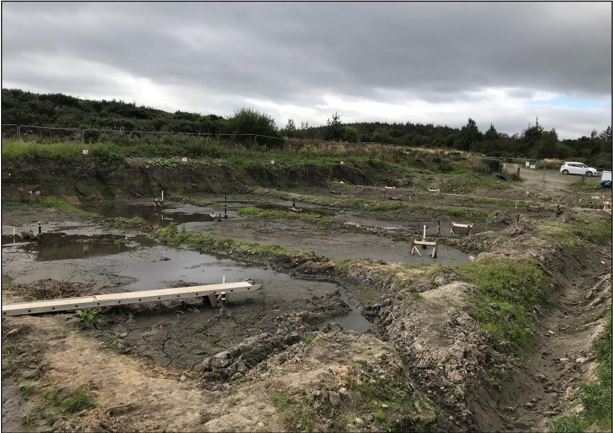
Figure 27. Deployment of Youngman board to access MW5 in cell F2.
