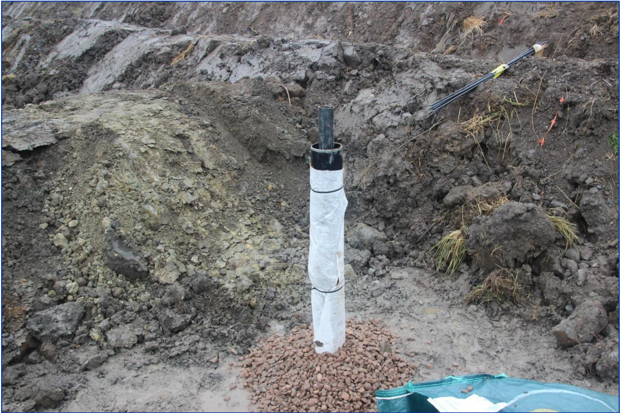
Figure 21. Construction of monitoring well/piezometers.
