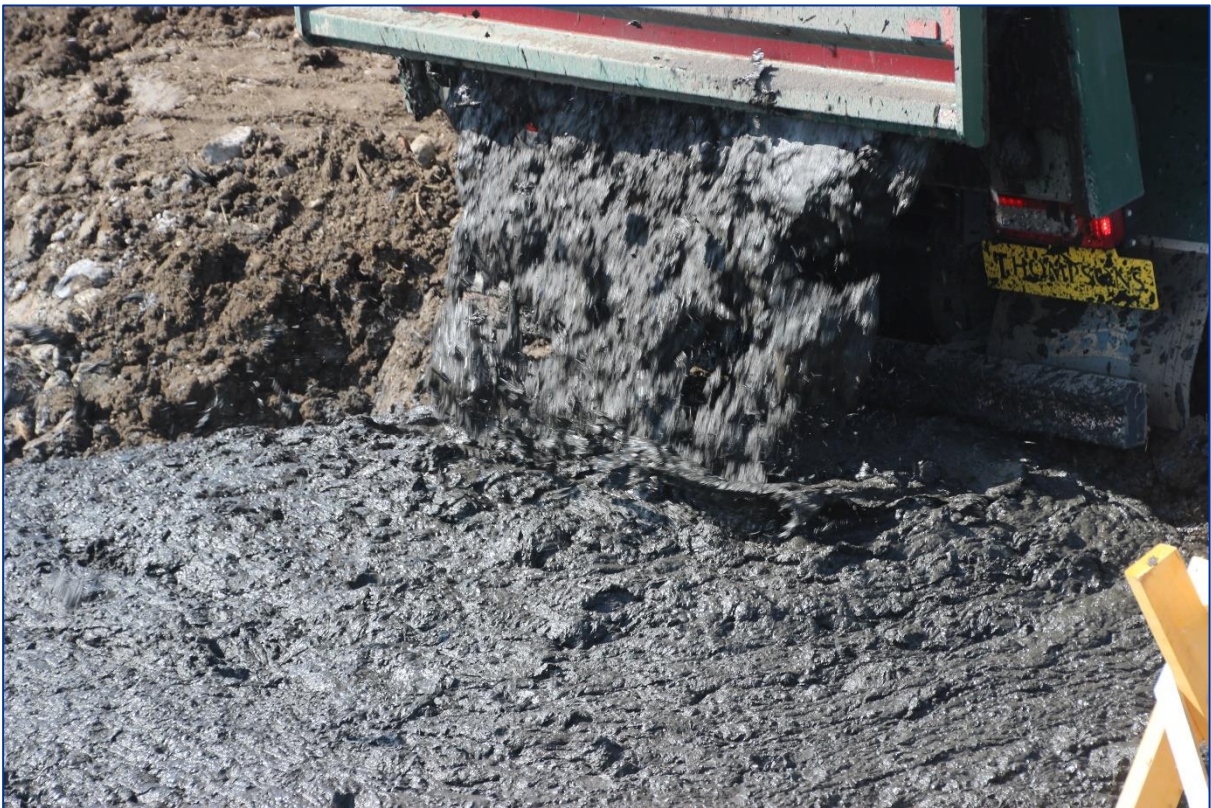
Figure 36. Sediment slurry being emplaced by tipper lorry.
