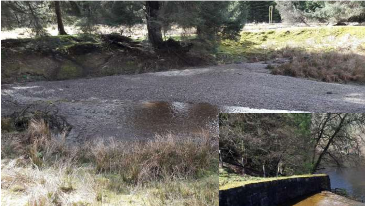
‘sediment’ trap with gravel
